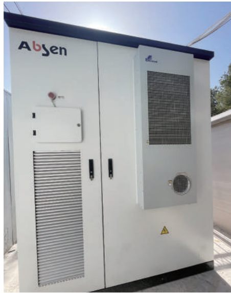
100kW/215kWh Middel East
